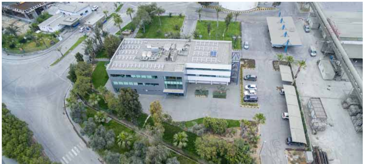
Panoramic view of the building and outdoors
