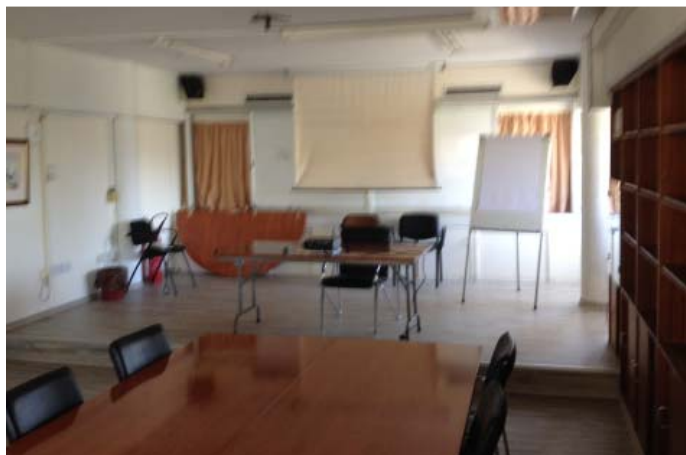
Interior areas Before Construction Work
