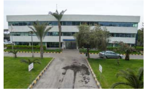
North View of the building after construction work
