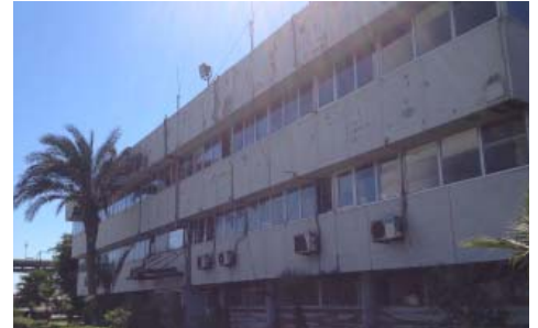
North View of the building before construction work
