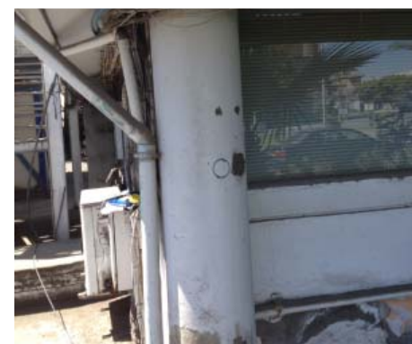
Exterior Building View before Construction Works.
