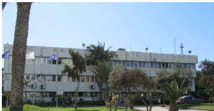
North View of the building before construction work
