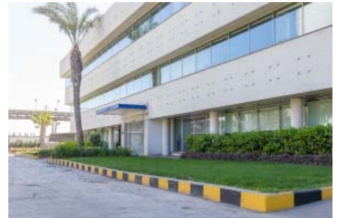
North View of the building after construction work
